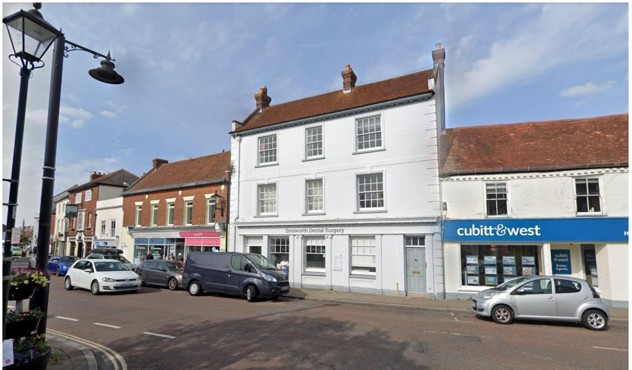
Figure 1: Front Elevation of Emsworth Dental Surgery on High Street.
