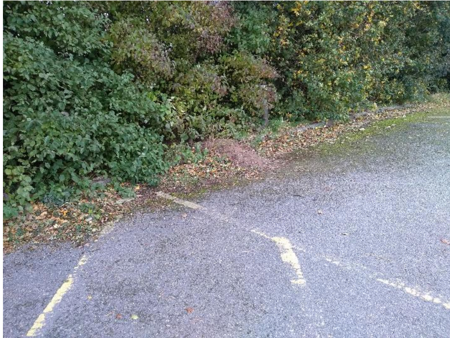
Figure 7: Image of dirt overflowing onto hardstanding due to sett digging
