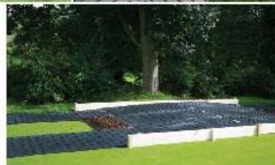
Ground-Guard trackways may be used with a cushion of woodchips to protect tree roots
