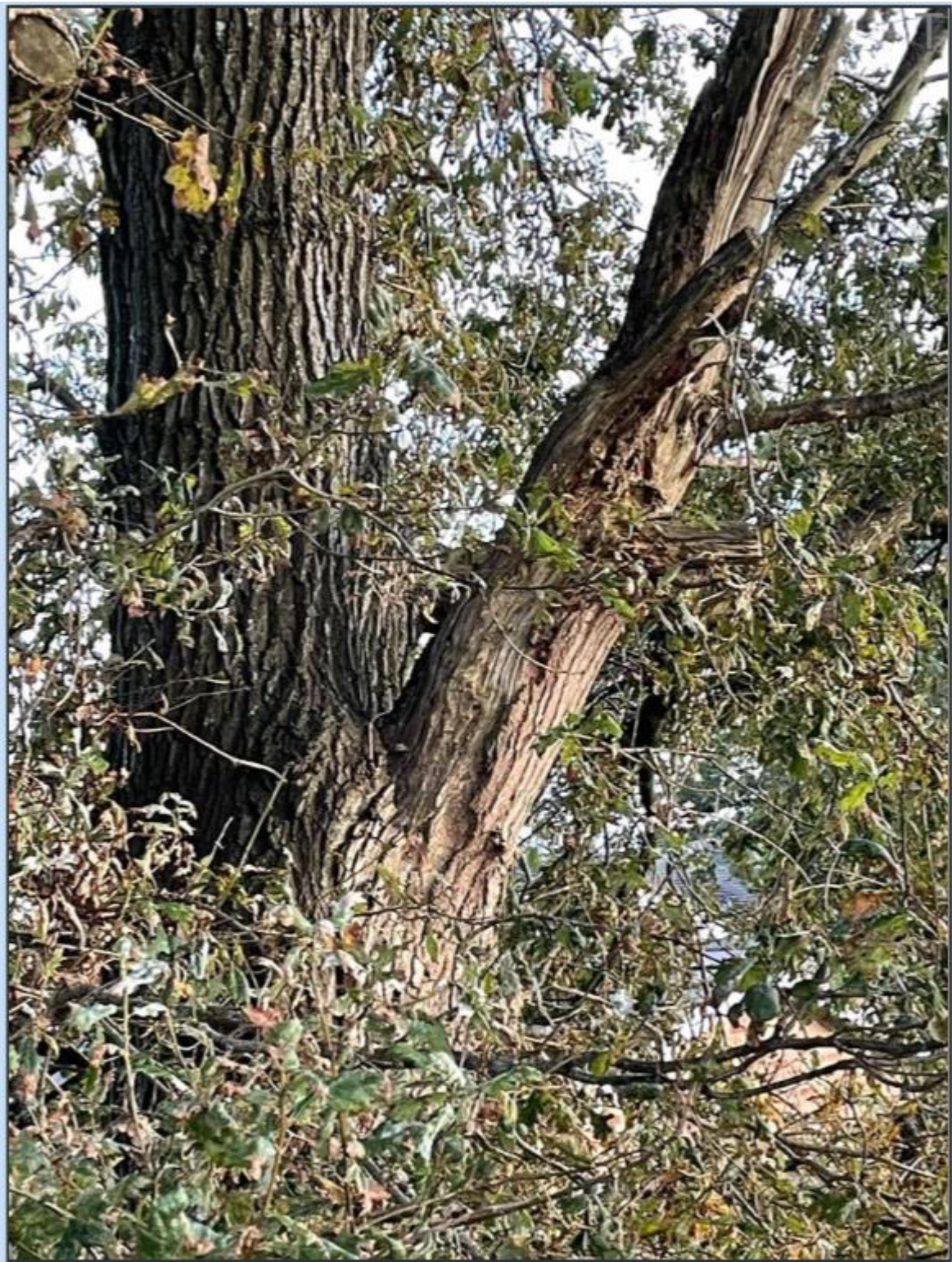
T4 previous failure on opposite stem
