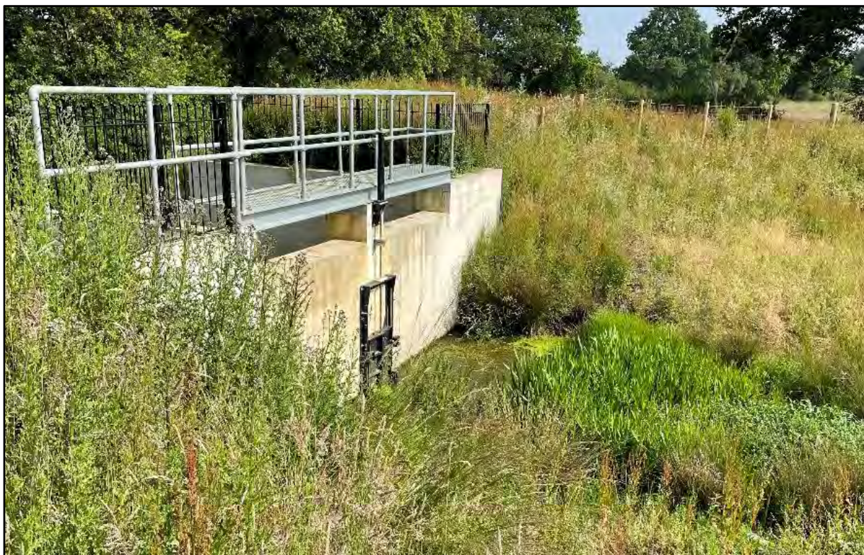
Figure 2-6: Flood attenuation area control structure (02/07/2021)
