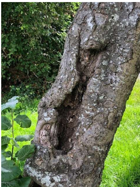
Photo 9. Stem decay evident to tree no.6
