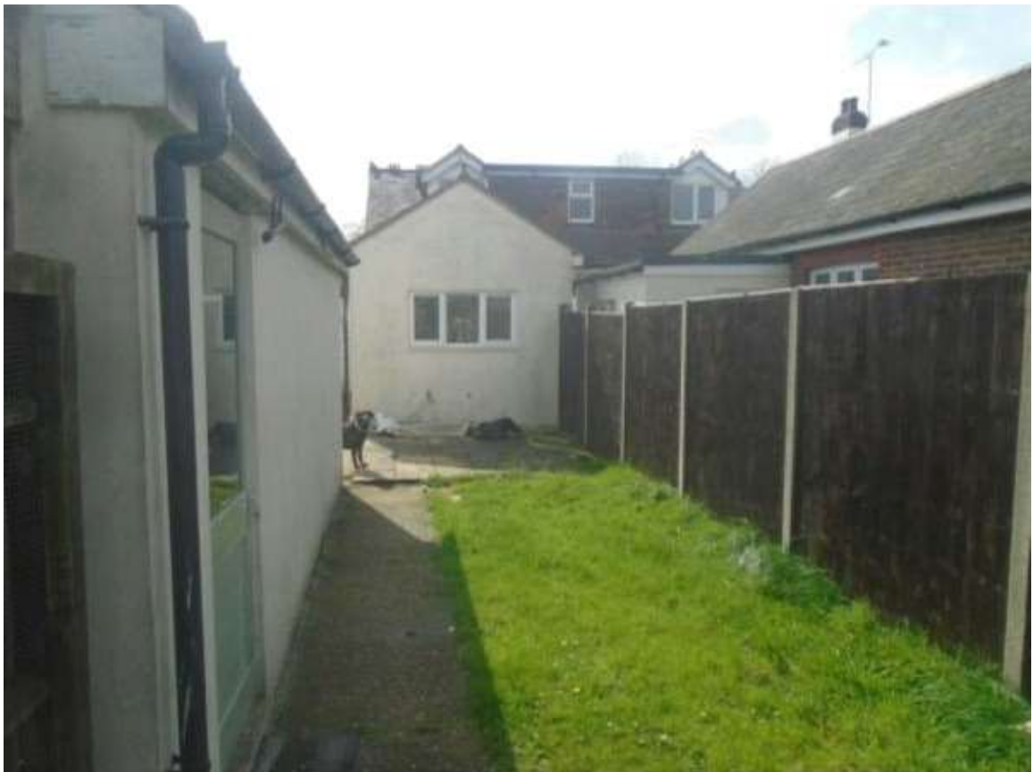
Figure 2. Rear of application dwelling and relationship with No.74A.
