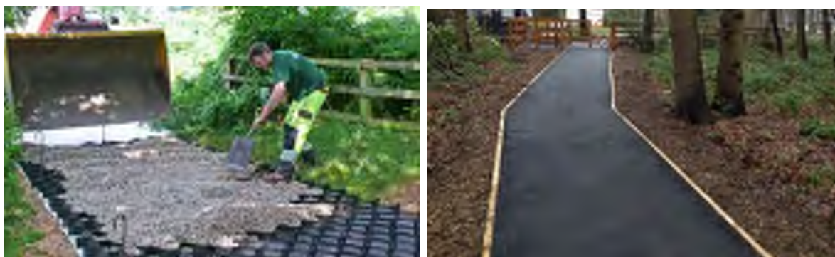
Figure 3.2: Root Protection System Example.
