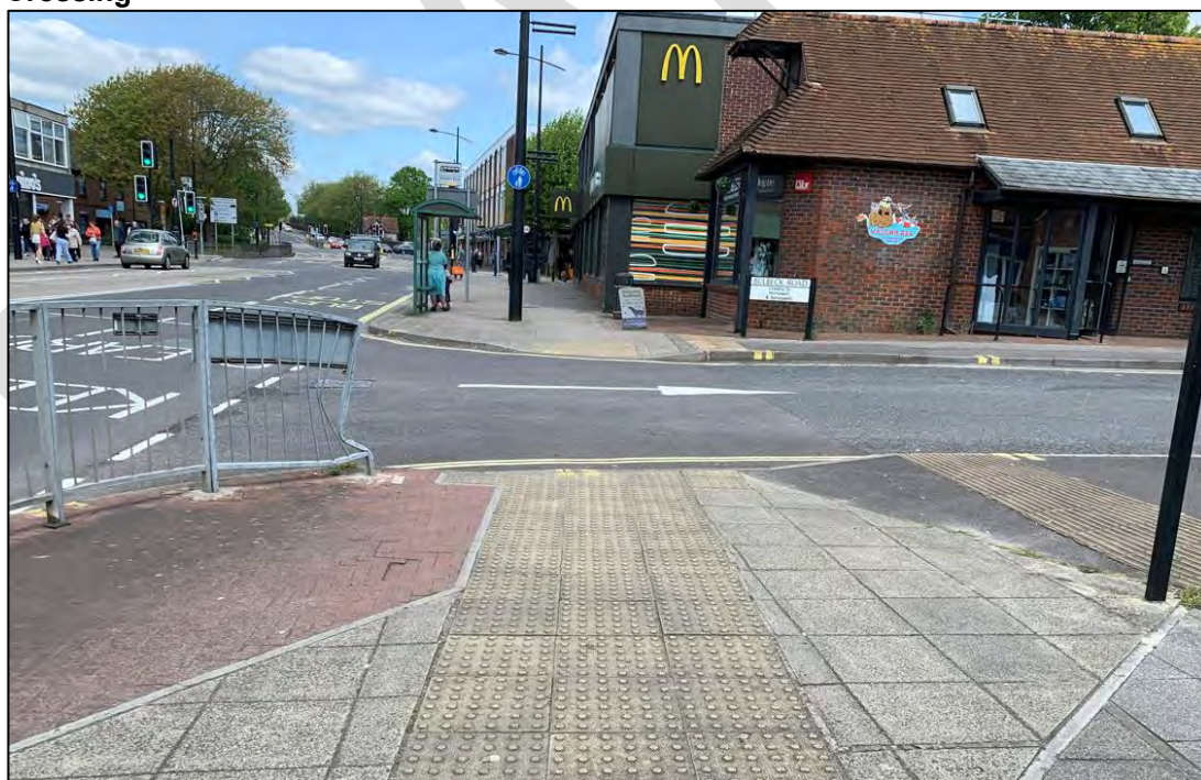
Image 2.9: Cycle Route Towards Havant High Street With Dropped Kerb and Tactile Crossing
