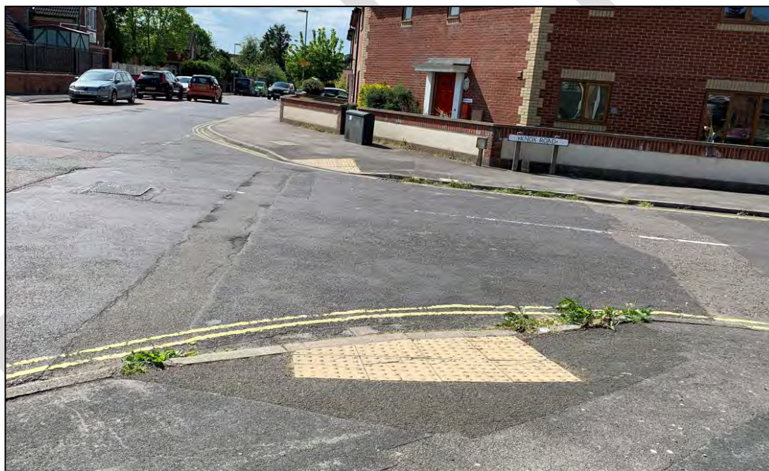
Image 2.7: Existing Dropped Kerb Tactile Crossing Across Knox Road (Eastern End)
