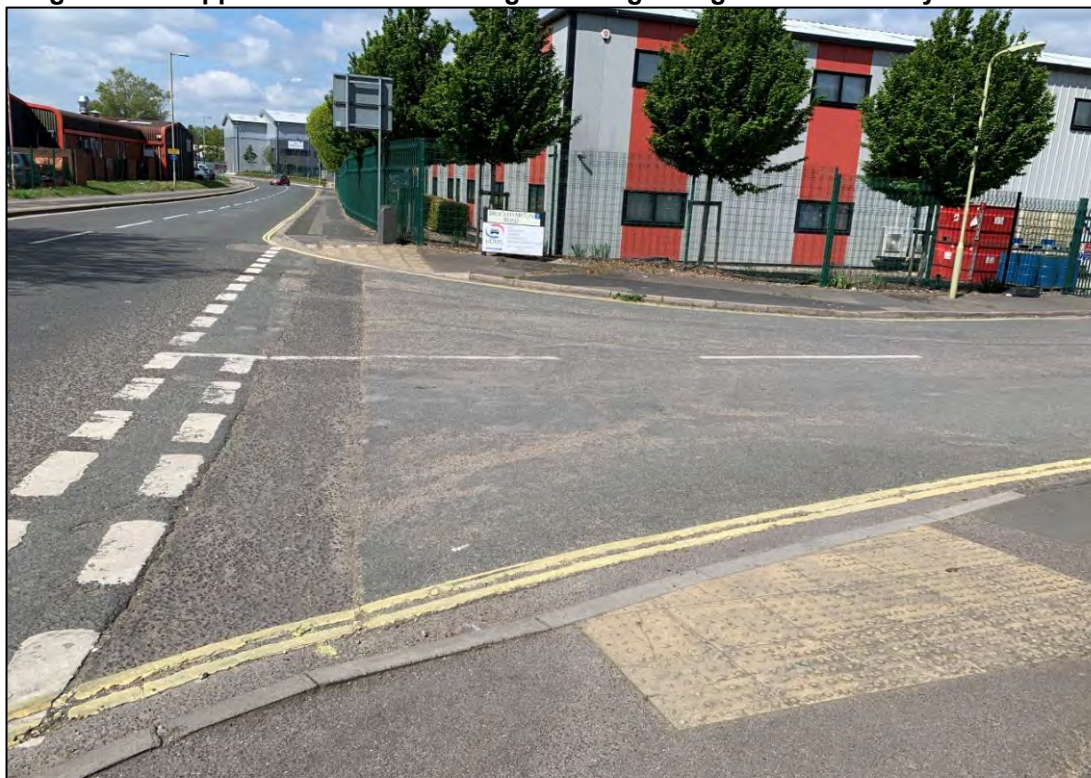
Image 2.12: Dropped Kerb Tactile Paving Crossing Along Harts Farm Way
