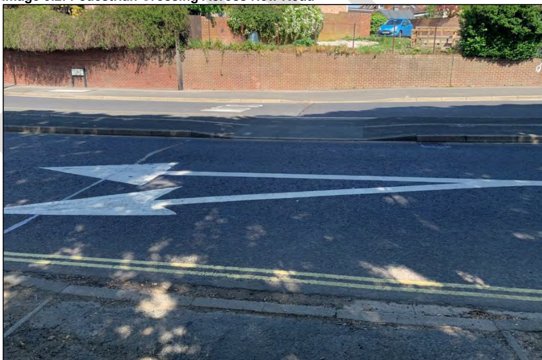
Image 3.2: Pedestrian Crossing Across New Road
