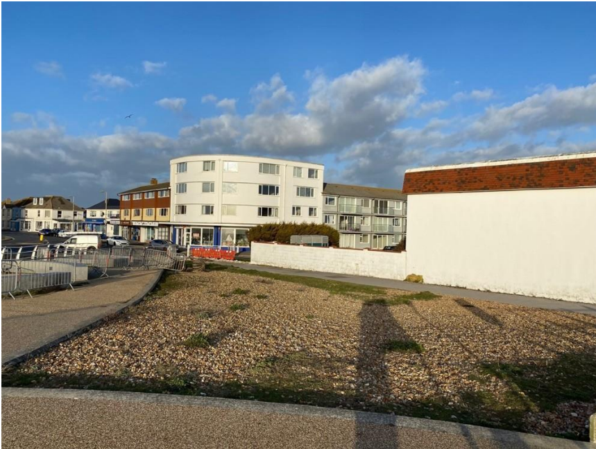
Looking Northeast from the footpath leading to the beach towards 2 Bembridge Drive and the flats opposite. The impact of the proposal is clear. Photo 2.
