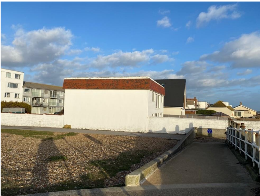
Looking East from the footpath to the beach with [redacted text] with the dark roof. Photo 3.
