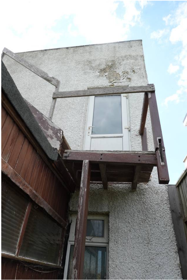
Photo 13 - View above Photo 12 showing rear first floor door and stair up to roof terrace.
