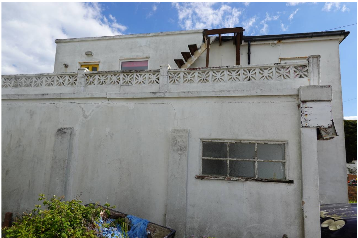
Photo 10 – View of north elevation to No. 29 facing towards the site..
