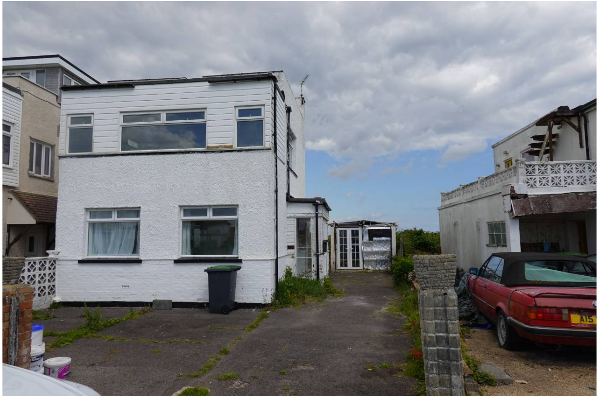
Photo 1 –View of house looking east from the road. No.24 just seen on left, No. 29 to the right..
