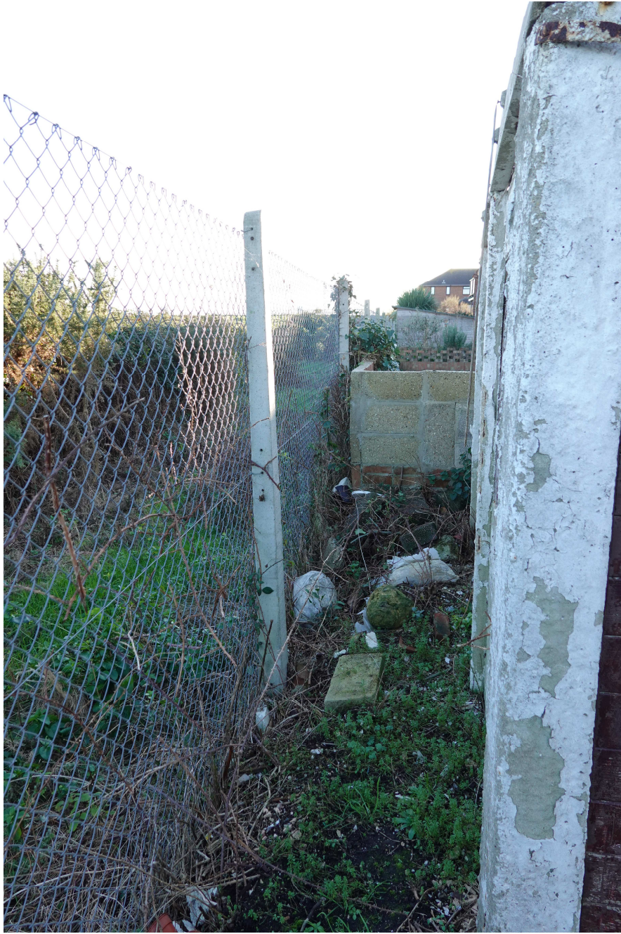
Photo 17 - View looking south-east towards back of garage to No. 25 and east boundary fence.
