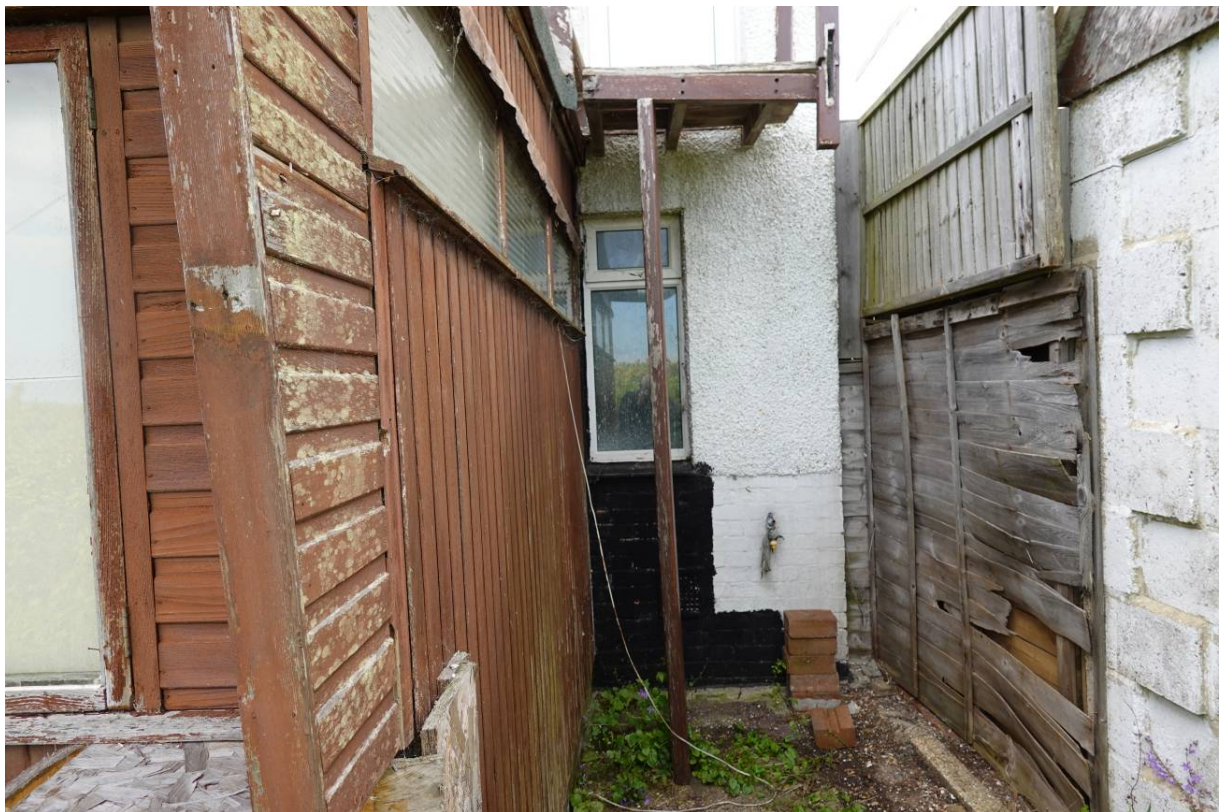
Photo 12 – View looking towards rear of No. 25 with north boundary to the right.
