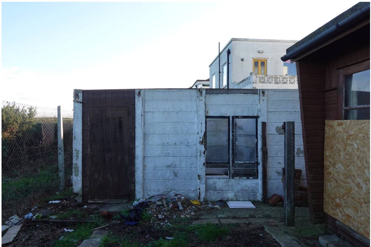
Photo 16 - View looking towards side of garage to No. 25 with No. 29 visible beyond.
