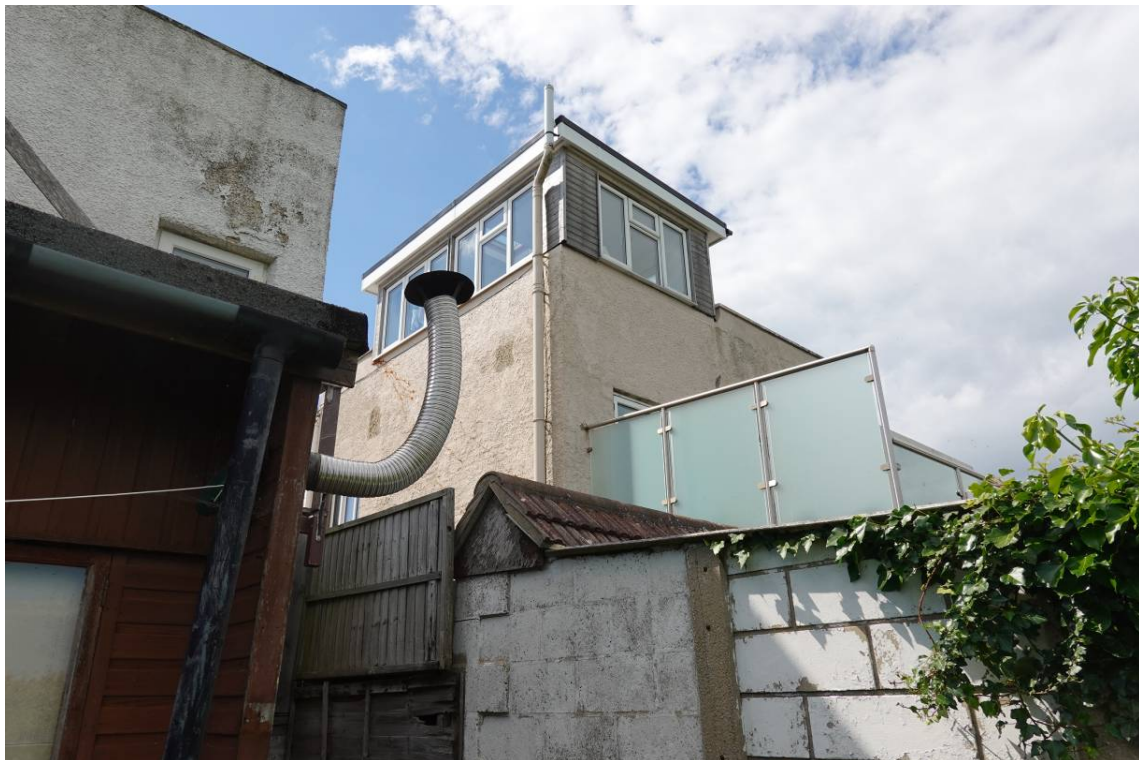
Photo 14 - View looking up towards rear of No. 24 with privacy screen to first floor terrace right of centre.
