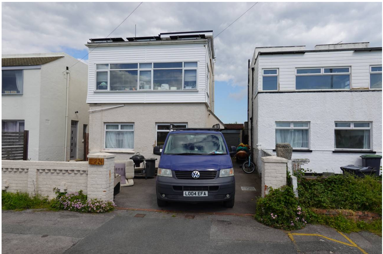
Photo 2 – View of No. 24 looking east with No. 25 to the right.
