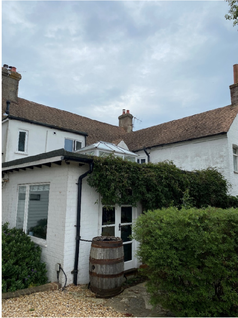
Fig.8 Lantern in the existing kitchen to be removed.
