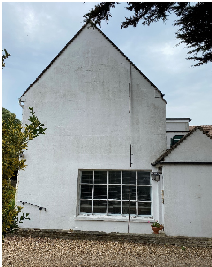
Fig.2 North façade of C18 house and modern bay entrance to the right.
