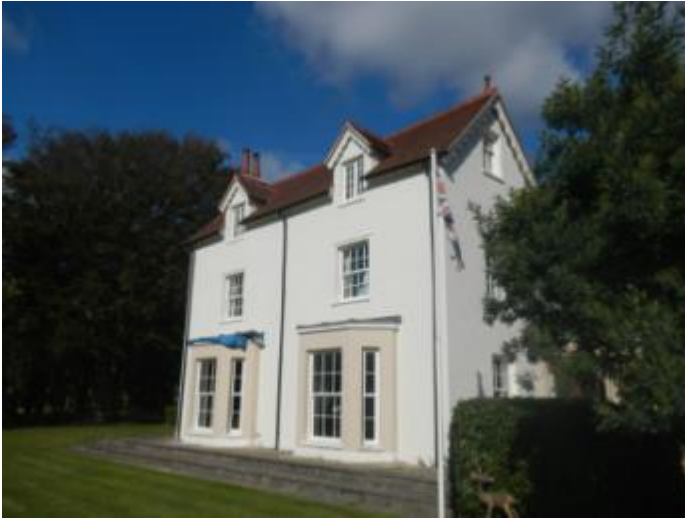
S elevation (unaffected by works)
