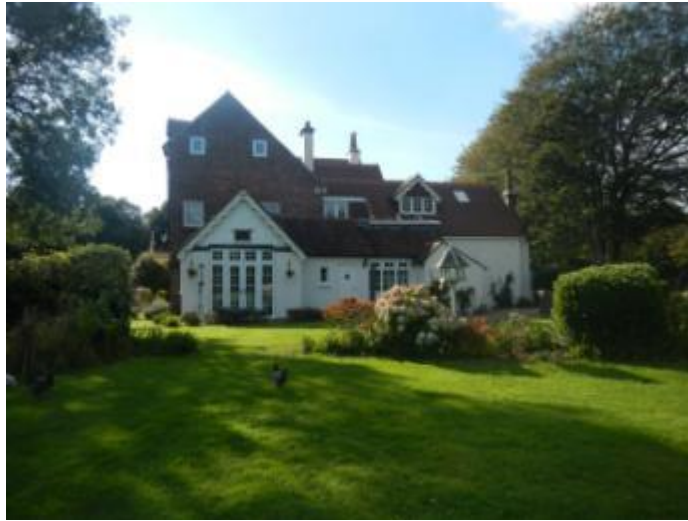
East elevation, single storey structures
