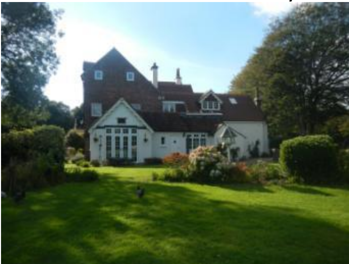
East elevation, single storey structures
