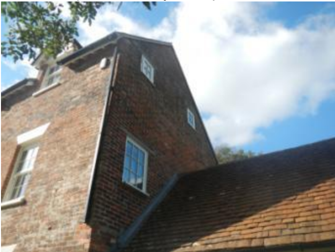
Interface of East elevation with the 3 storey main building, not tiles intact.
