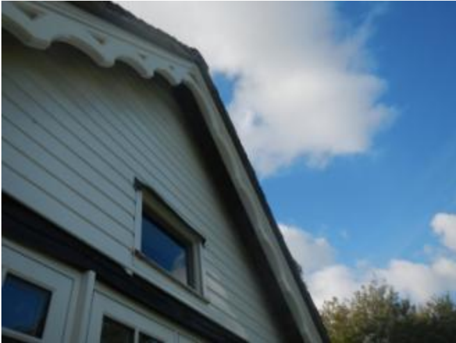
Detail of recent wood boarding to single storey structure
