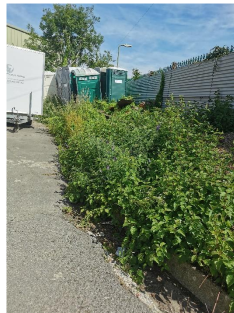
Ruderal present at northern elevation of building
