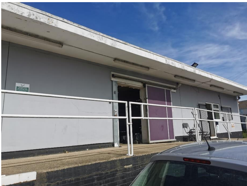
South-eastern facing elevation of main building showing degraded building and lack of roosting features
