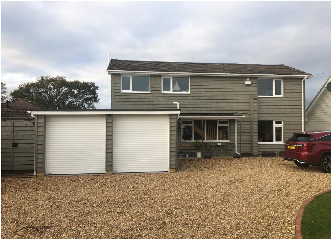
51 North Shore Road – Front view
