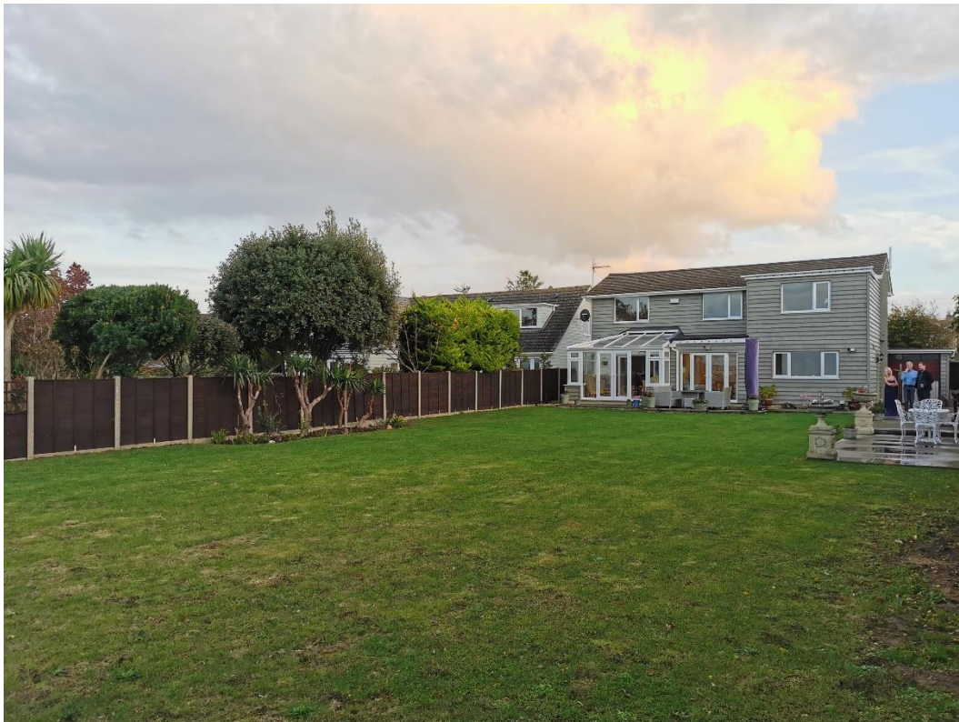
51 North Shore Road – Rear view
