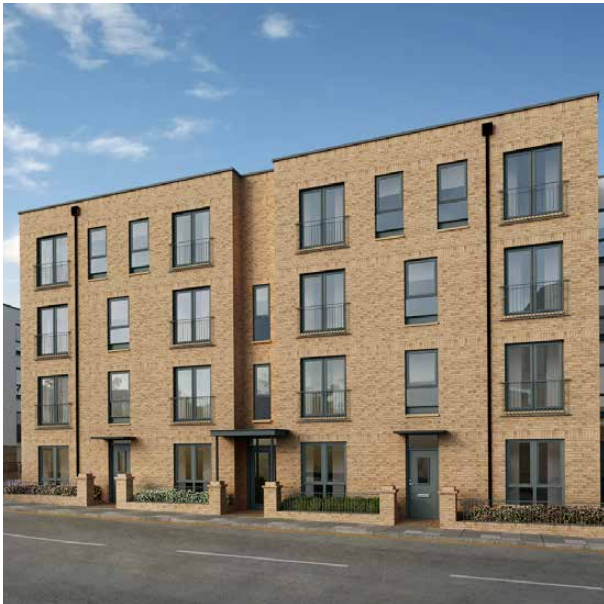
Apartment block in buff brick With stepped elevation highlighting the entrance
