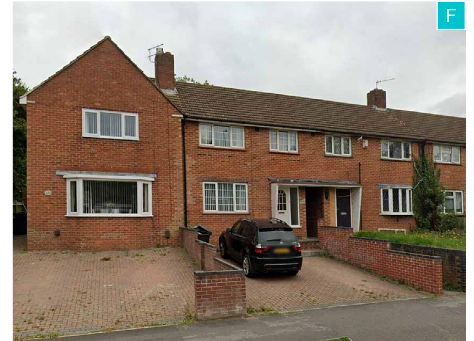
Orange Brick Houses on Dunsbury Way
