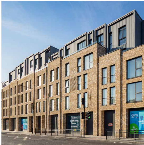
Mixed use block in buff brick With zinc top floors
