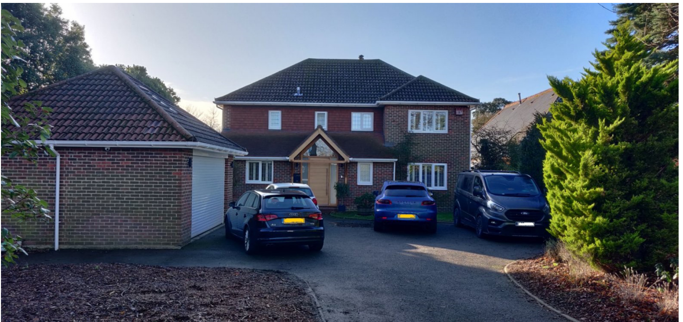
Front elevation 30 Hollow Lane showing existing garage to the left of photo.
