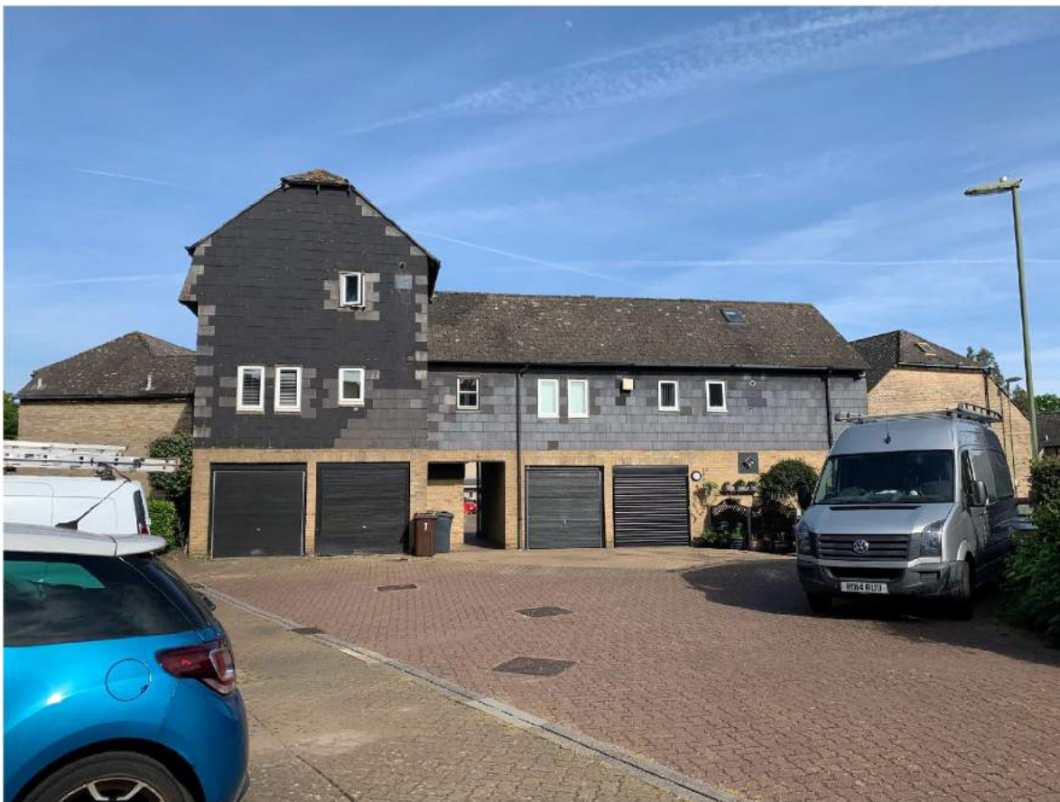
Rear facade - Existing
