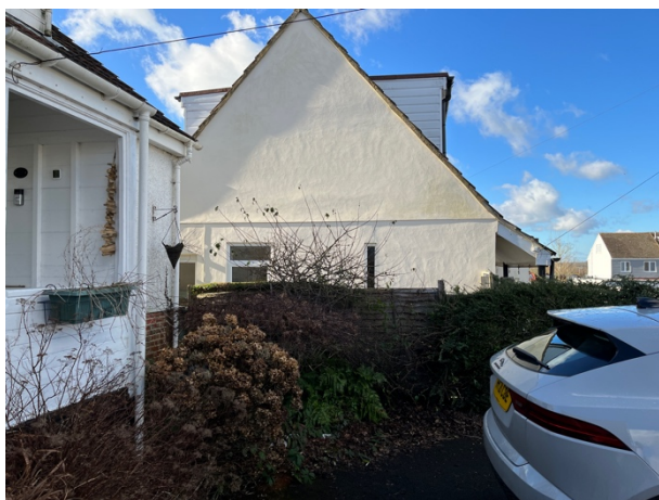
The side (east) elevation of no.2 Privett Road, next-door to the west of the application site.
