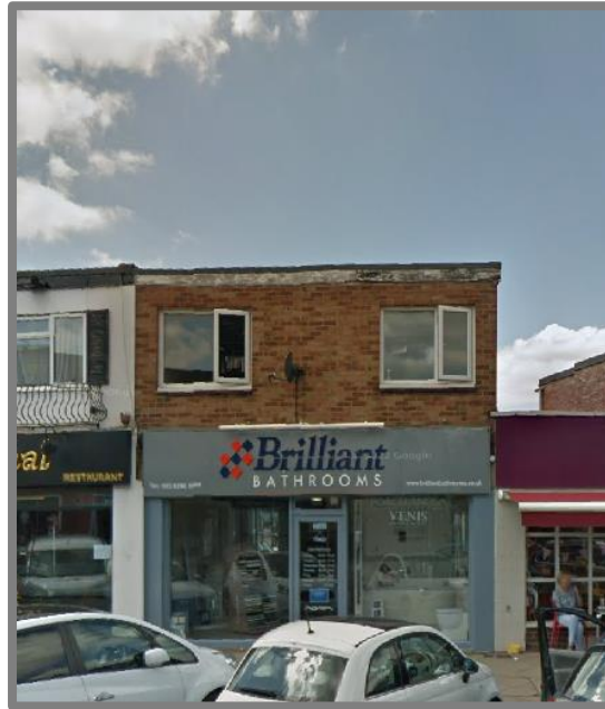
Figure 1: Front elevation of 53a Station Road
