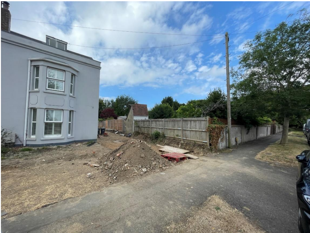
Site Viewed from outside 57 Park Road
