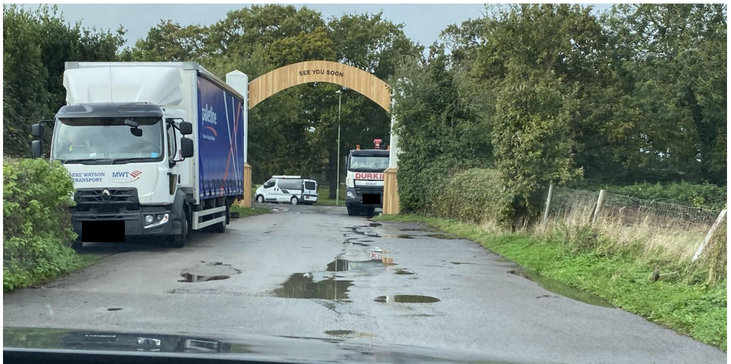
Fig 44: Source: TWE photograph.
