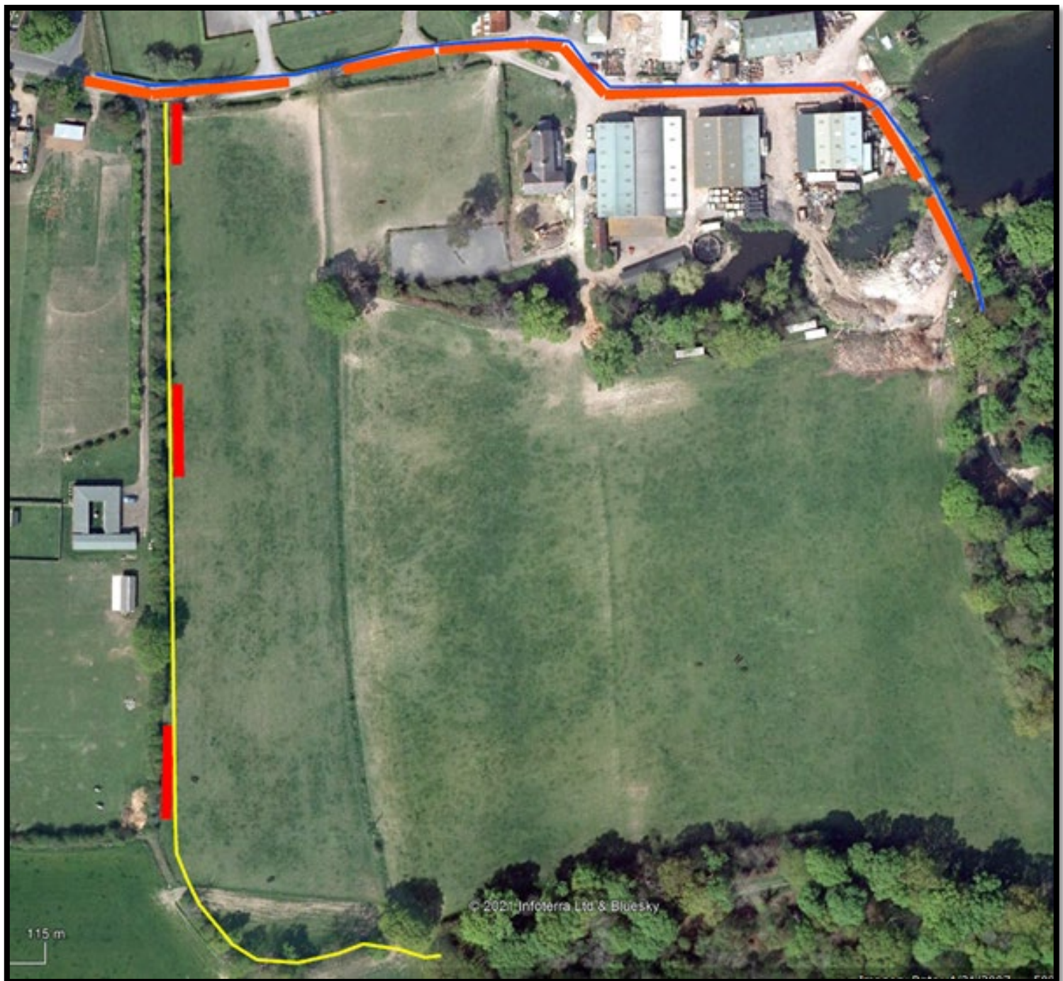
Fig 8A: Source: Google Earth image. The blue line shows the existing Right of Way and orange lines show distances where the Right of Way on the ground is usable to over 4.5 meters in width. The yellow line shows the new alternative access (as granted planning permission in 2017 & granted again with variations in October 2021) and the red lines show where this alternative access is more than 4.5 meters wide, which is only two 30 meter long passing places and the first approx. 20 meter entrance splay.
