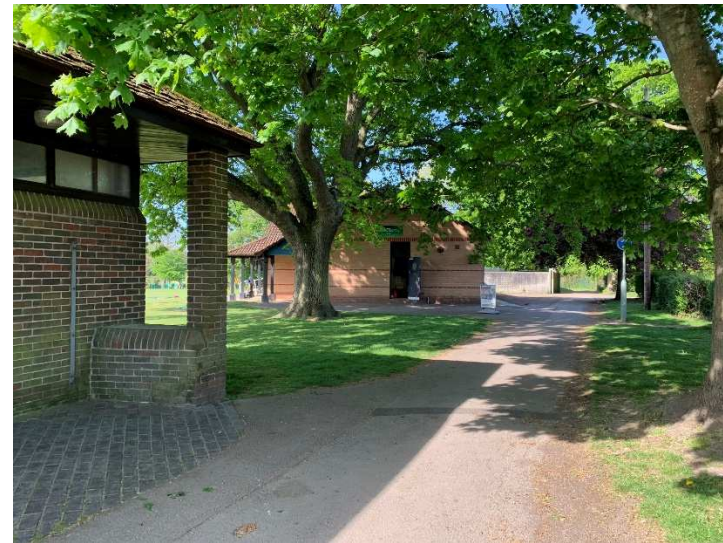
East elevation of pavilion when approached from car park
