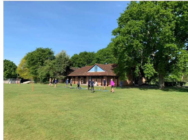
South elevation of existing pavilion
