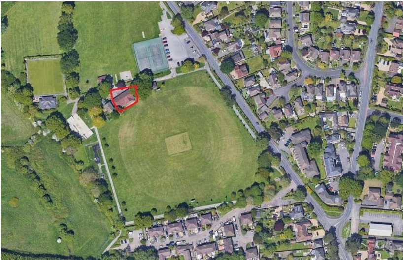
Aerial photo of site showing pavilion (Google maps)
