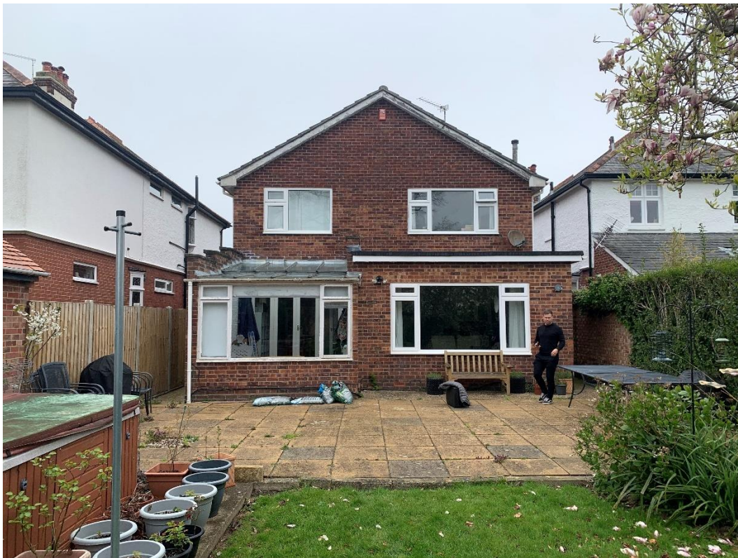
Rear of 10 Langstone Avenue.
