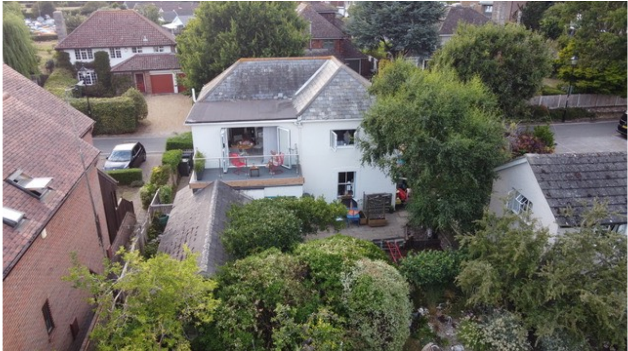
Rear elevation and setting as existing
