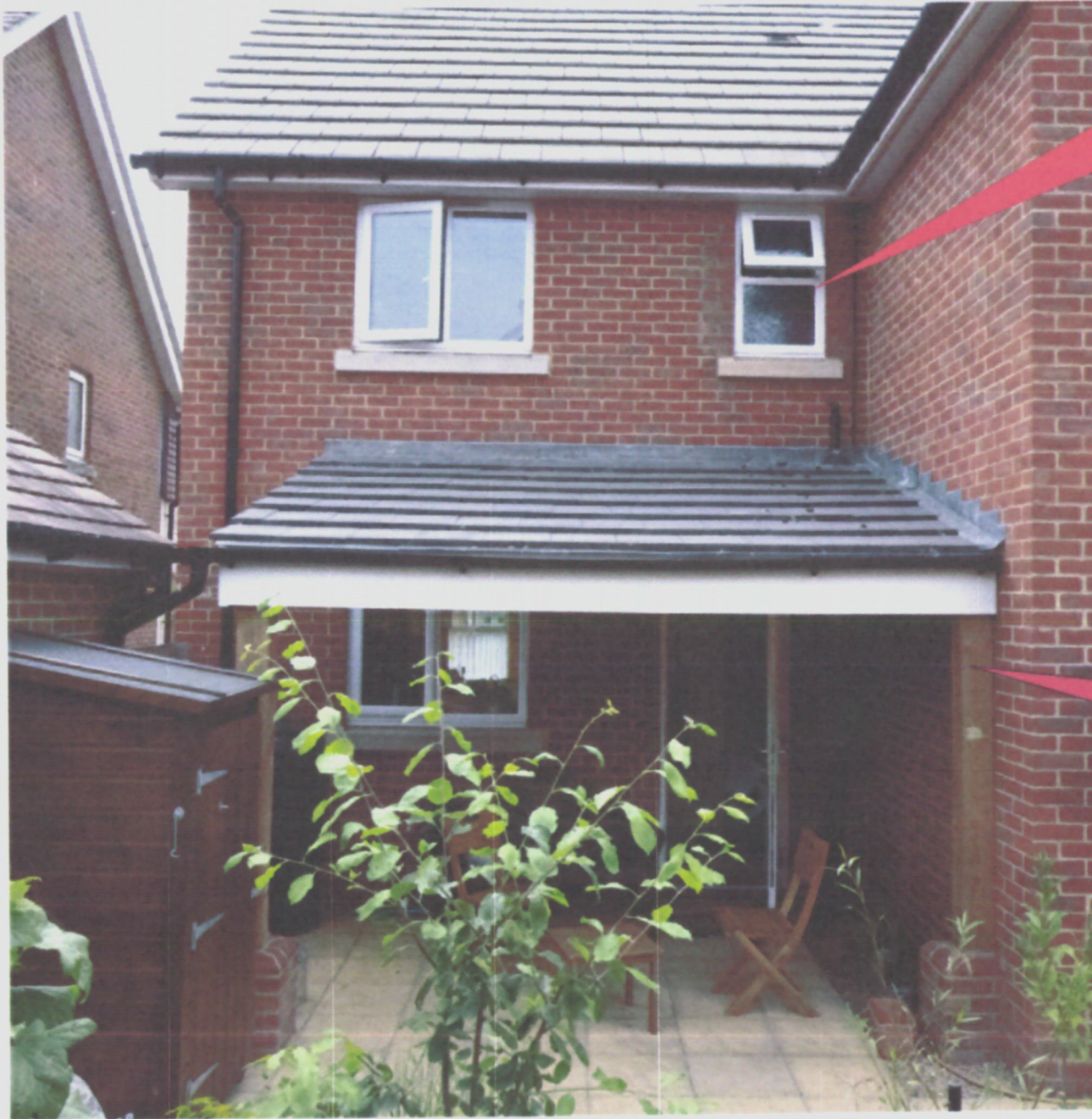
Photo 1: Rear of house
