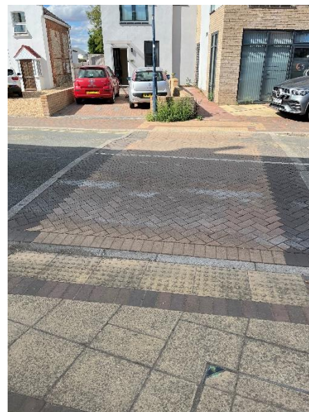
Photograph 6: Pedestrian crossing point on Station Road
