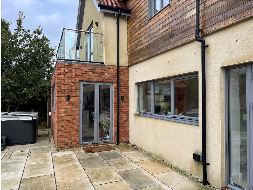
Figure 7: Existing Rear Elevation [Location of Proposed Rear Extension]
