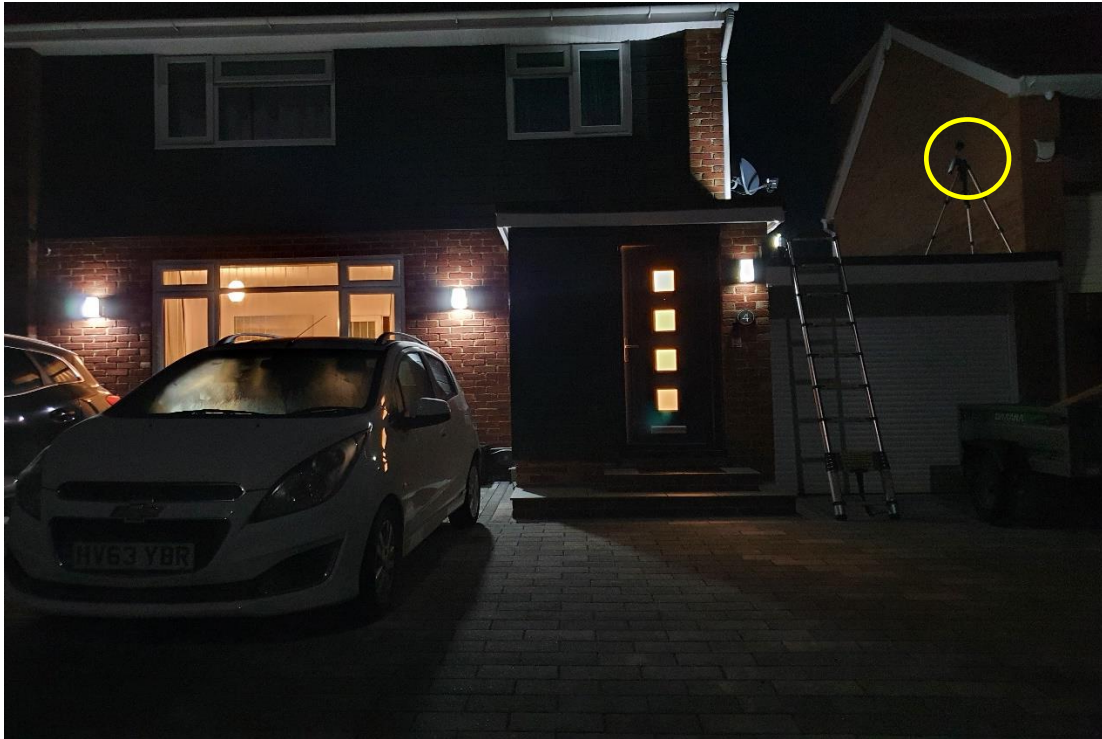
Photo 3 Measurement location 2; on garage roof
