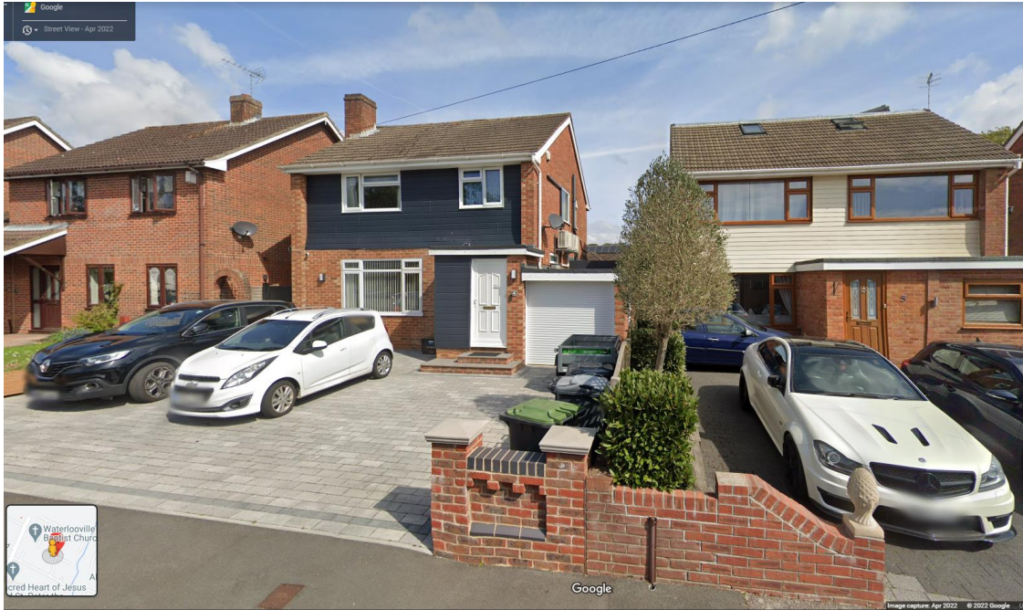
Photo 1 4 Bramley Close, two A/C units are visible above the garage
