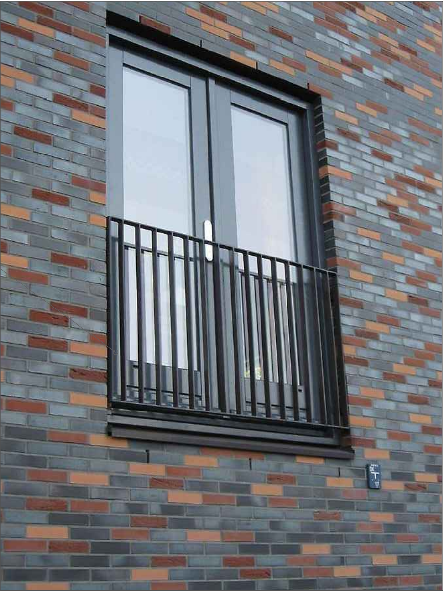
Metal railings juliet balcony
