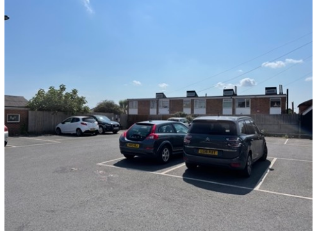
View of rear of the terrace from South Street Carpark
