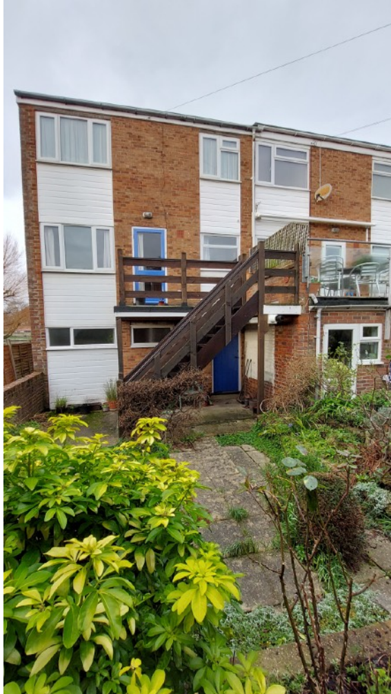
View of rear of the property
