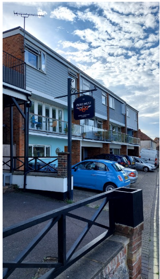
View of front of the terrace showing variation in elevational treatment
