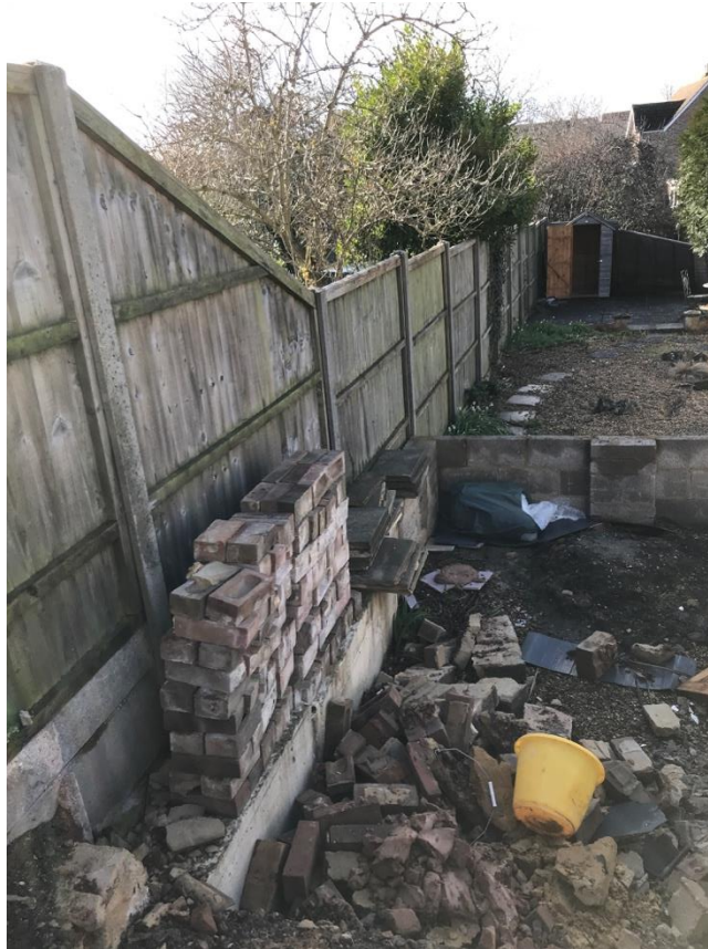
View looking down the garden, the new walls partially built for the proposed additional terrace.
