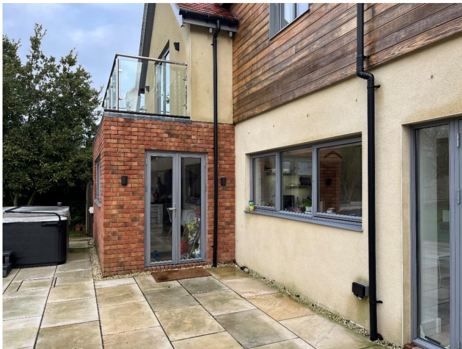
Figure 2: Existing Rear Elevation [Location of Proposed Rear Extension]
