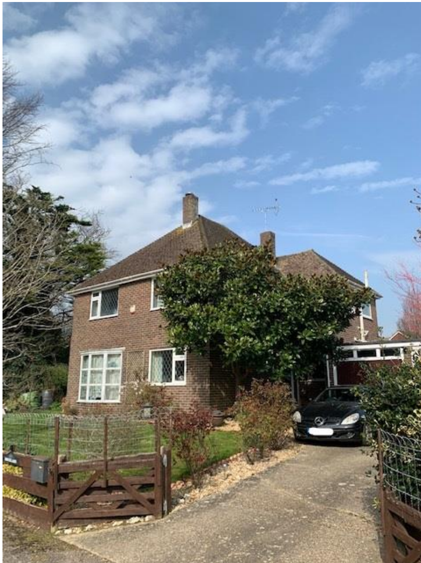
Figure 1: Image of Front of Existing Property. Taken by Applecore PDM
