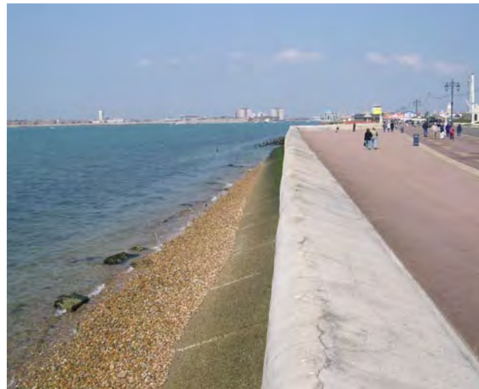
Sea wall at Southsea, Portsmouth.
