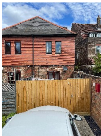
1 Chapmans Court (at centre, part of adjoined pair, house 2 at left) - view from street (Twittens Way cul-de-sac - current pedestrian approach). Twitten to right, beyond boundary wall.
