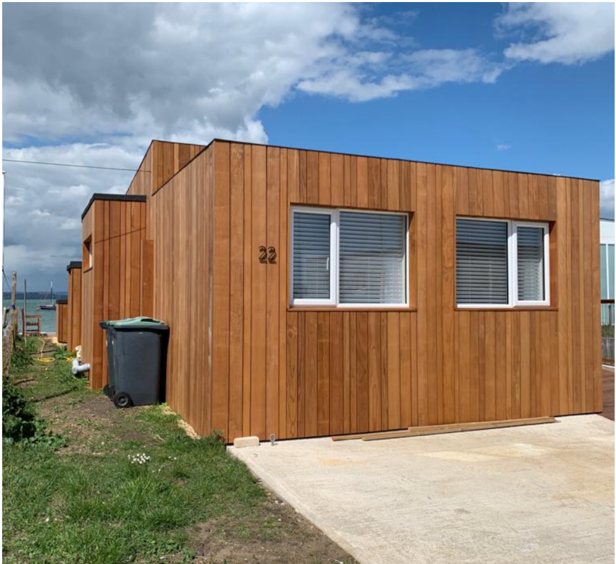
Photo 3: West elevation showing new wood cladding soon after fitting
