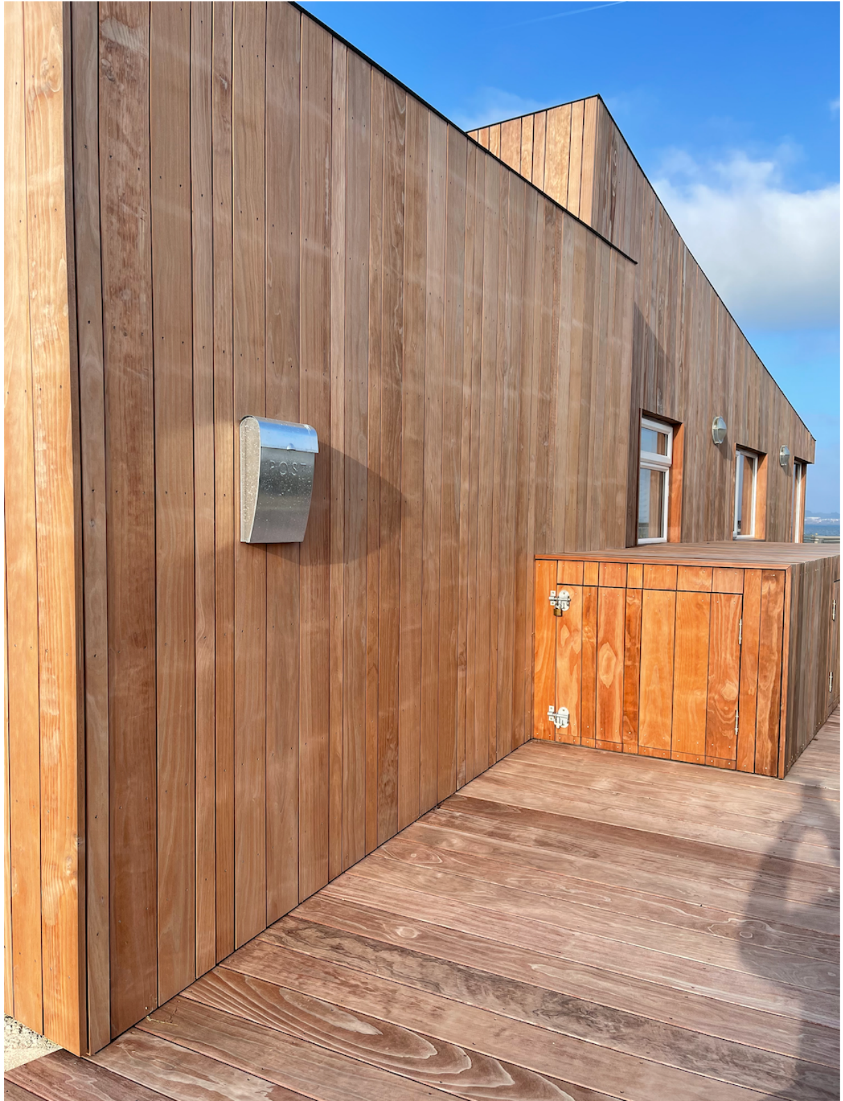
Photo 4: East elevation showing new wood cladding several months after installation. Wood is already fading and going silver. This process continues.
