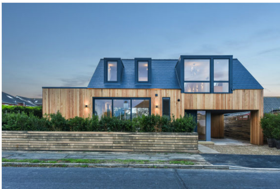
The Application Site No. 3 Nutbourne Road following development
