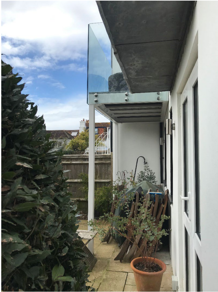
Plate VIII : Balcony at 5 Orange Row, viewed from Tower House. The revised balcony design will be very similar appearance to this.
