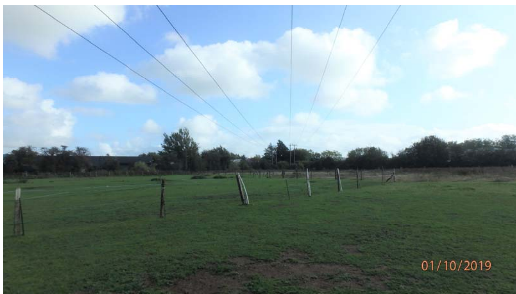
Plate 4 – View from northern pylons, following line of power cables looking south east
