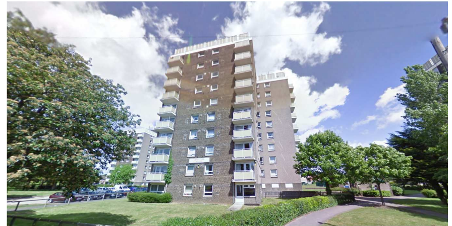
Existing view of Langstone House from Lockerley Road [Google Maps]
