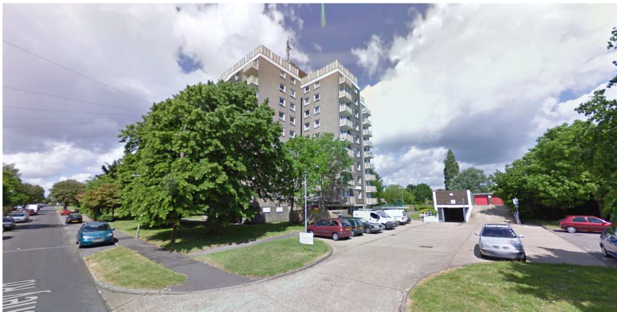
Existing view of Chichester House and the existing two-storey garage from Lockerley Road [Google Maps]
