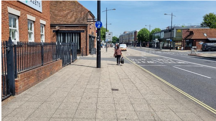
Photo 15: Looking north on Park Road South
