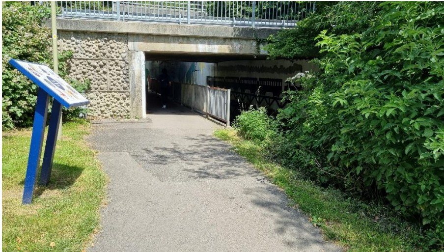
Photo 1: Looking north towards the southern underpass
