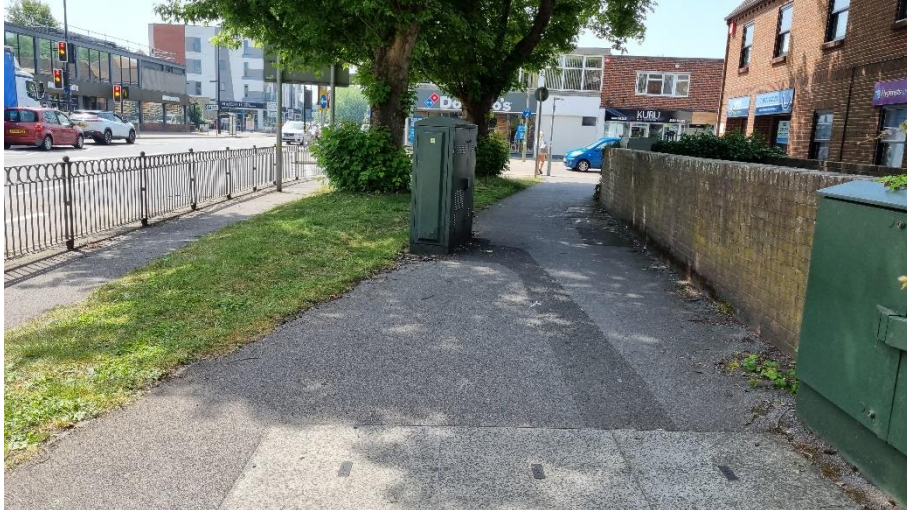
Photo 18: Looking south towards raised table crossing at West Street
