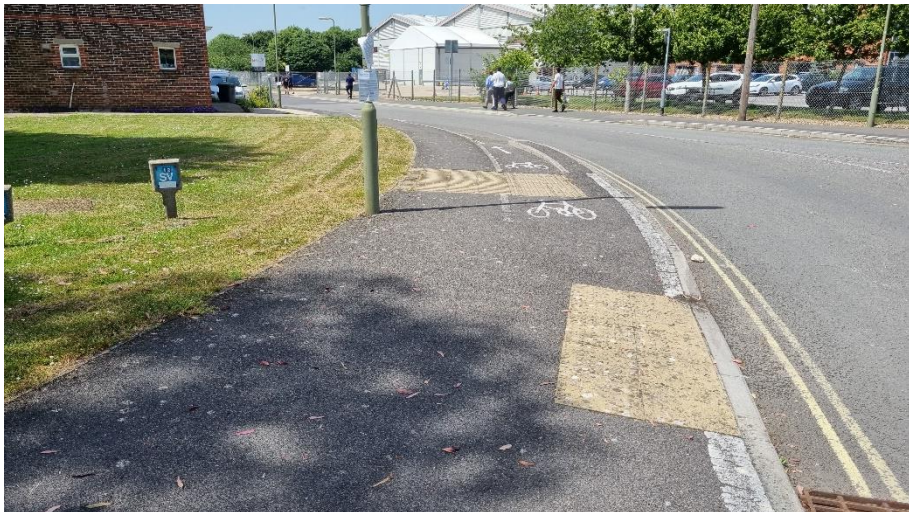
Photo 44: Looking west from the Brookside Road roundabout (southern side)
