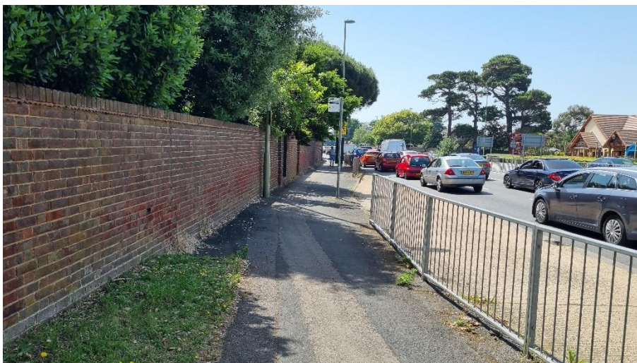
Photo 45: Looking south towards southbound bus stop on Langstone Road
