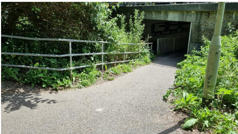
Photo 3: Looking south towards the northern underpass
