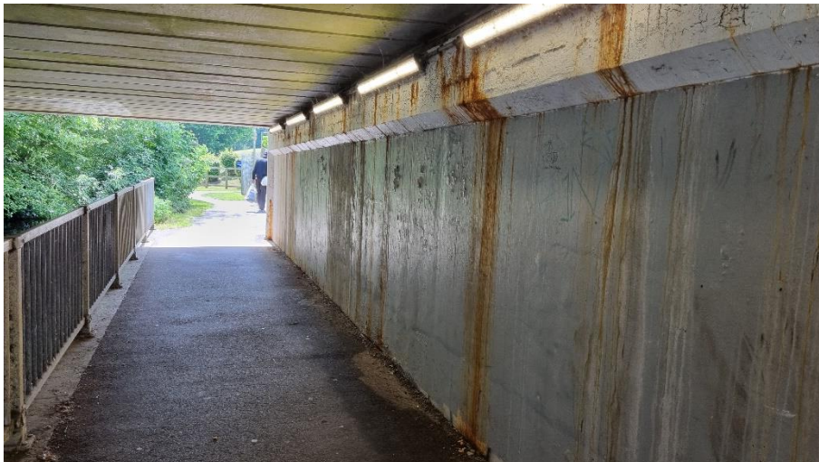
Photo 2: View from within the southern underpass
