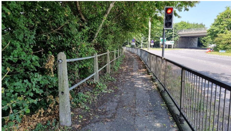
Photo 52: Looking northwest toward A27 westbound on slip at A27 junction
