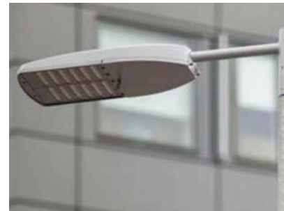
COLUMN LIGHTING TO SERVICE YARDS, ROADS AND CAR PARKING AREAS
