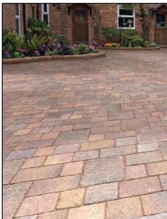
5. Concrete sett paving for approach to building
