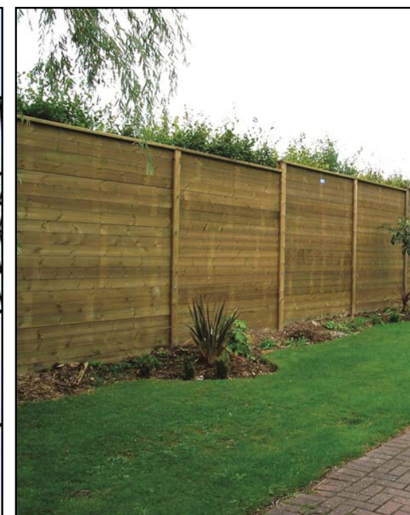
8. Acoustic Fence to deliveries area perimeter
