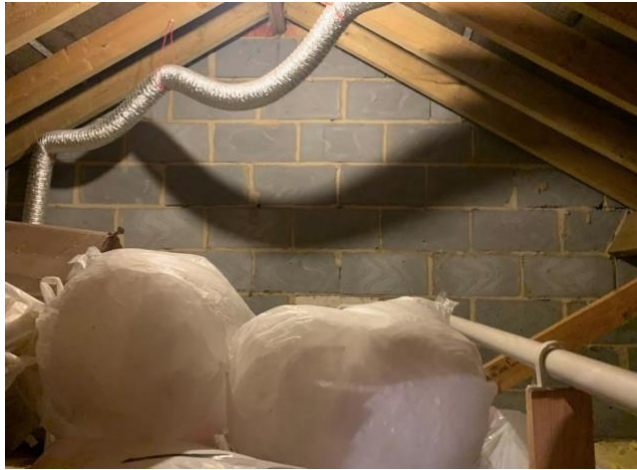
Figure 8. View of the loft space of No 65 with intact roofing felt underlining the tiles.
