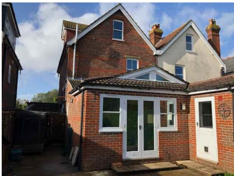
Existing rear extension – with low pitched roof
