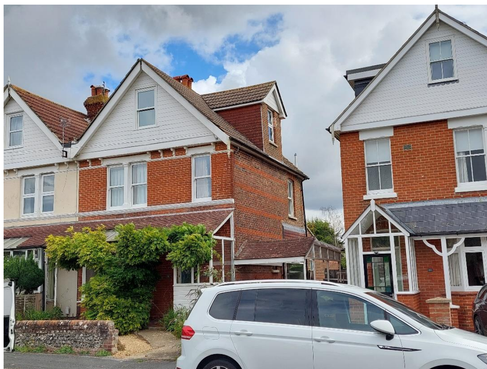
Existing Dormer to No.18
