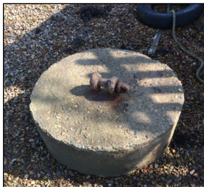
Figure 4: One of 14 mud mooring concrete blocks to be removed from the designated site.
