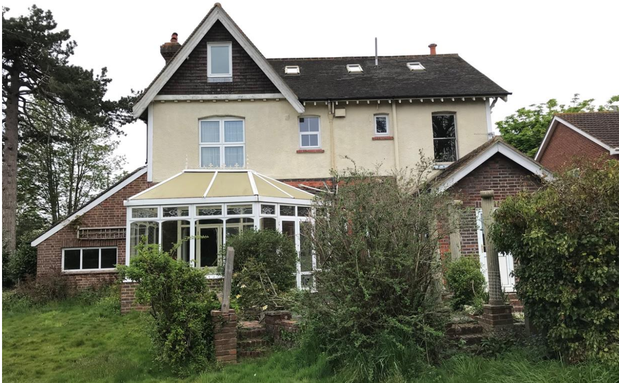
Figure 9 View of Dwellings Existing Rear Elevation
