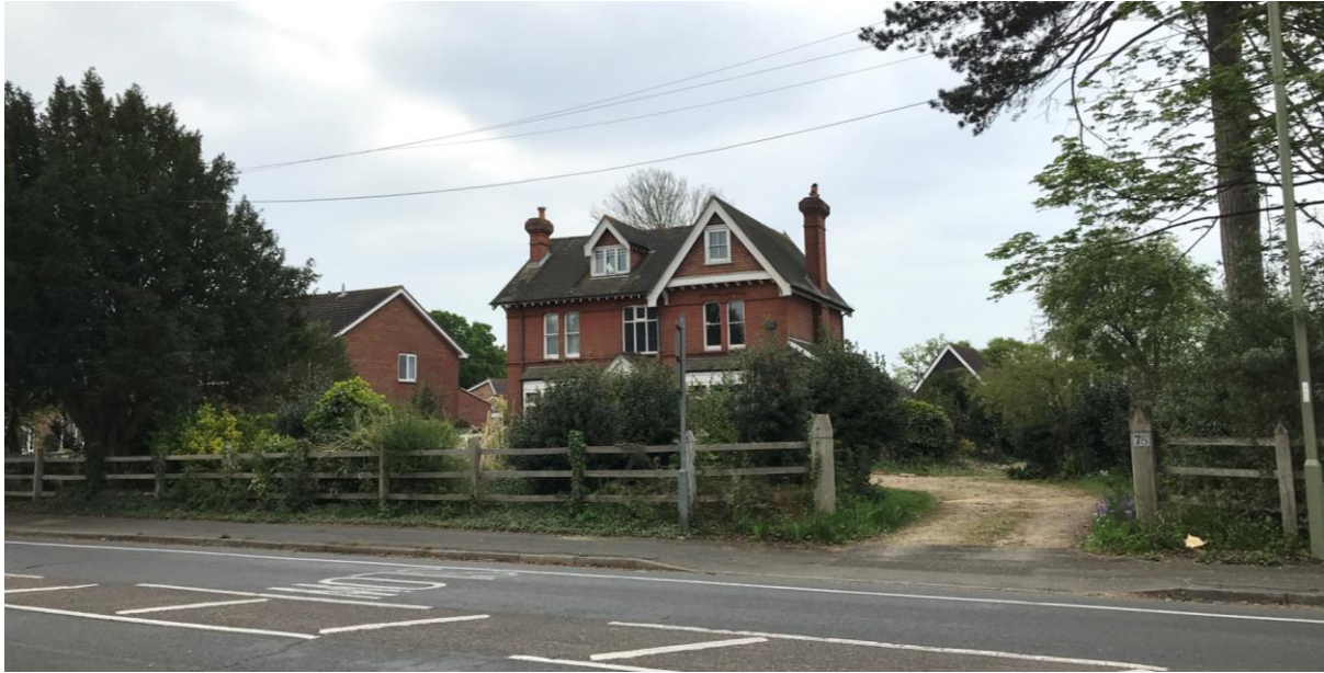
Figure 3 View of Application Building from Havant Road
