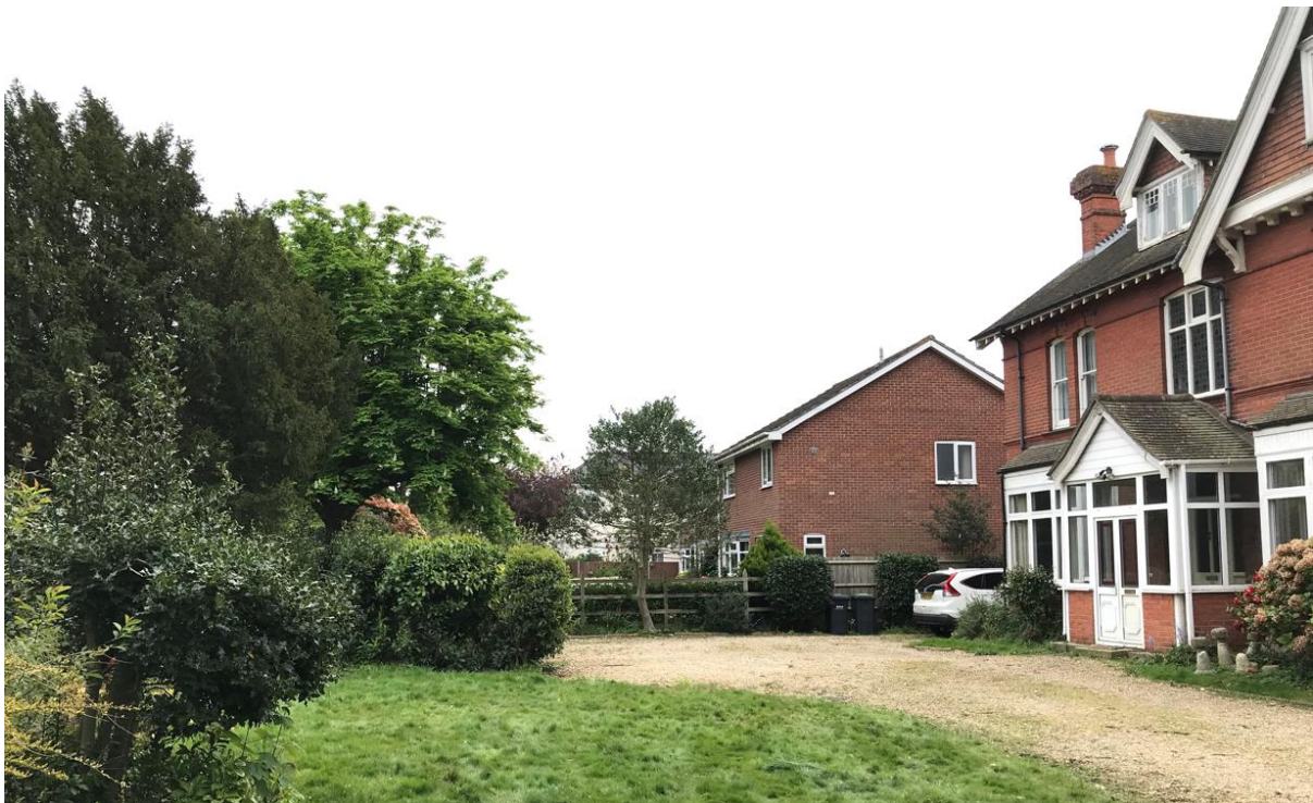
Figure 6 View Across Frontage of Existing Dwelling – West to East
