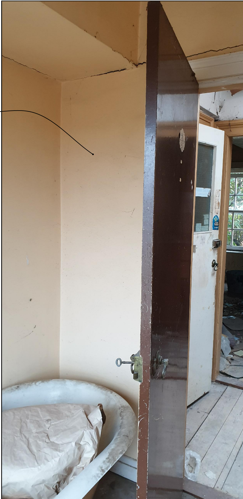
Bathroom looking towards Lobby
