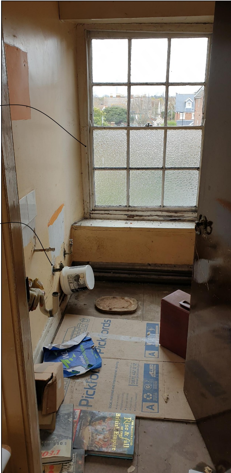
Bathroom looking South
