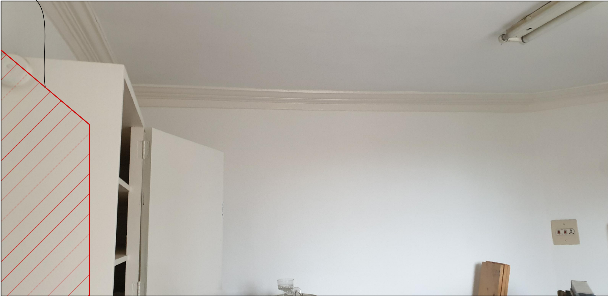
Southern Wall of Kitchen
