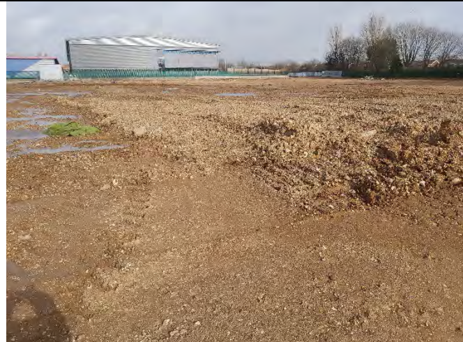
General view looking to northwest corner. Poned water following wet weather and storms on sacrificial layer.
