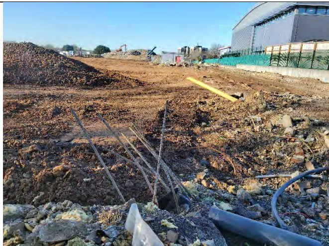
Western platform Class 2C rolled fill, completed.
