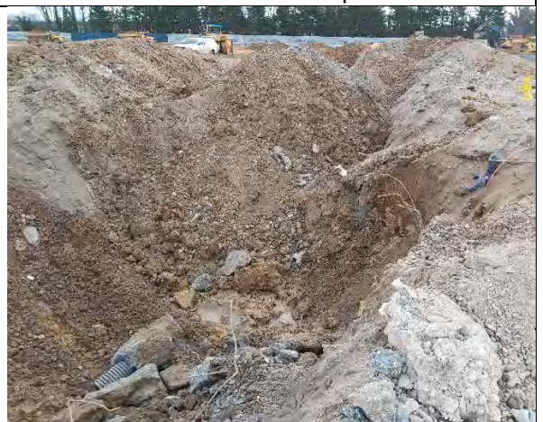
General view of deep concrete foundation excavation in southern area.
