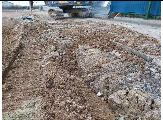
Excavation of concrete foundations eastern area of site.
