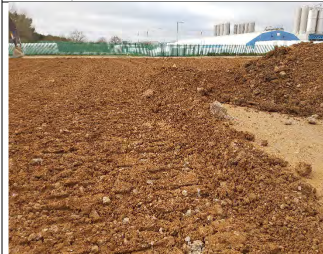
Fill prior to rolling.
