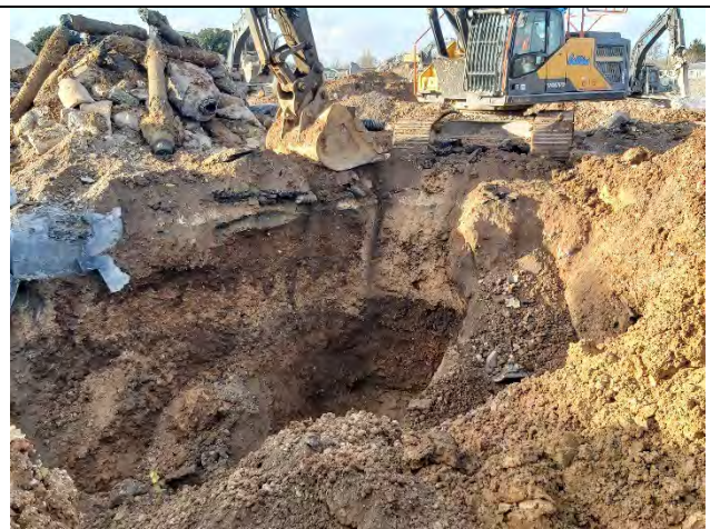
Excavation of reinforced concrete piles.
