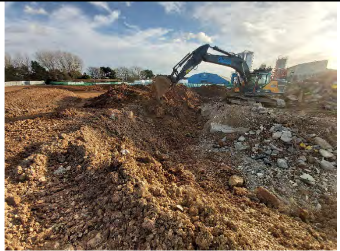
Excavation of concrete foundations in southern area of site.
