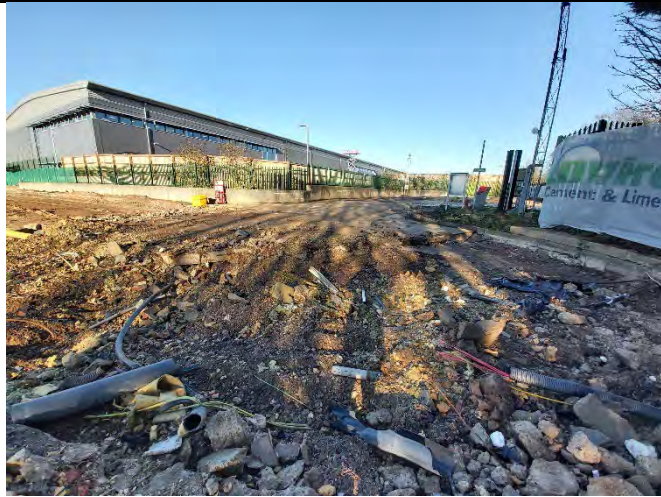
General view, northwest corner, incomplete.
