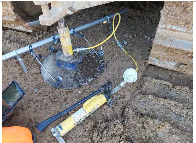
CBR plate load testing in central north area.
