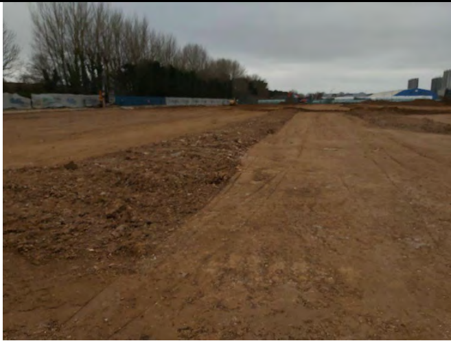
Northern strip completed to formation.
