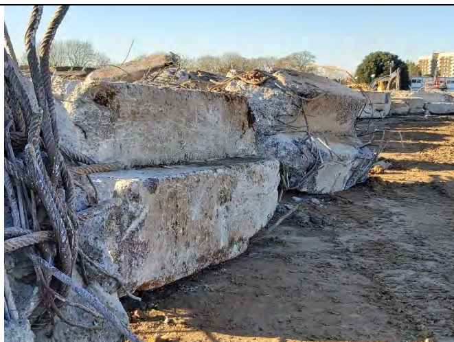
Concrete foundations excavated from eastern area.
