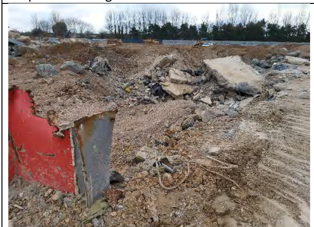
General view of deep concrete foundation excavation in southern area.
