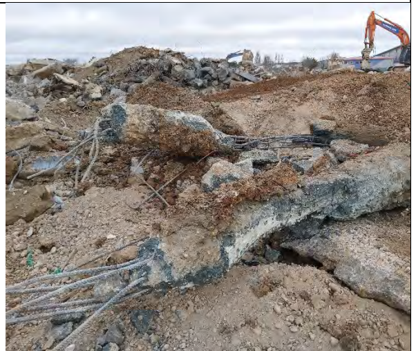
Excavated reinforced concrete piles.
