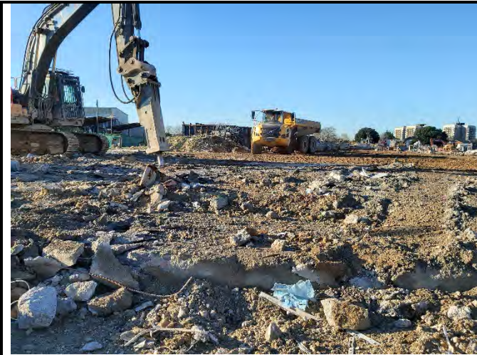
Breaking out concrete slab and substructures in eastern area.
