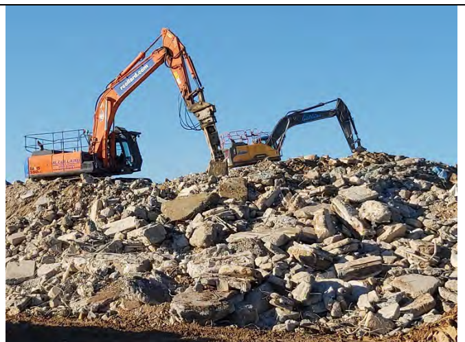
Concrete stockpiled for crushing.
