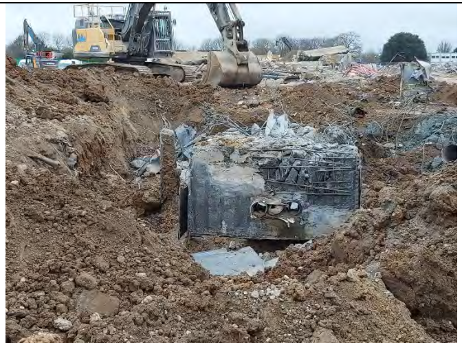
Excavation of concrete substructure.
