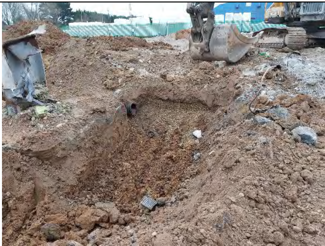
Head Gravel in excavation beneath Made Ground.
