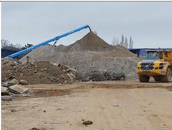
Crushing concrete, Class 6F5.
