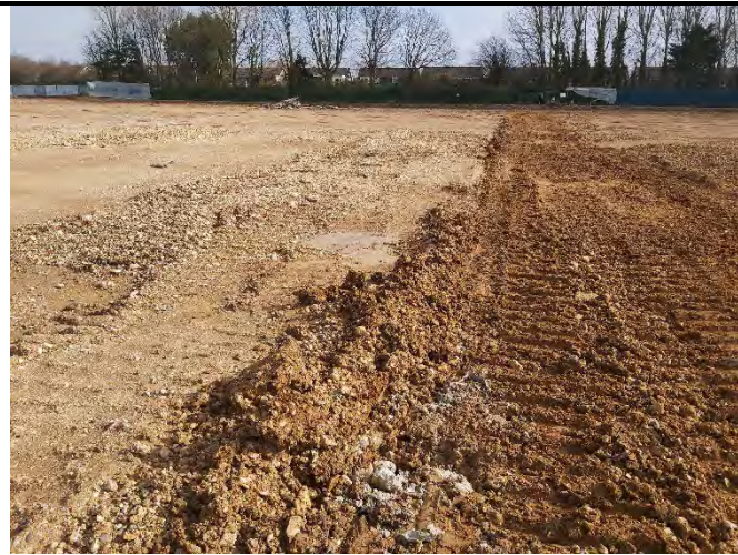
General view, looking north, incomplected fill to east of building footprint.
