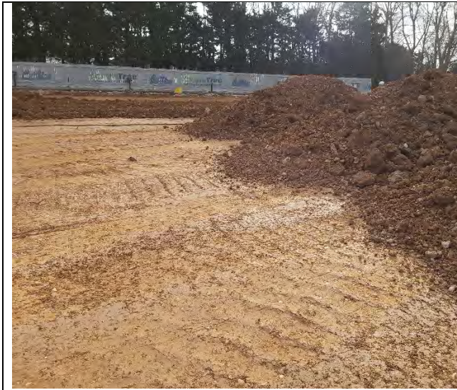
Rolled formation surface in south east area of site with stockpiled Class 2C.
