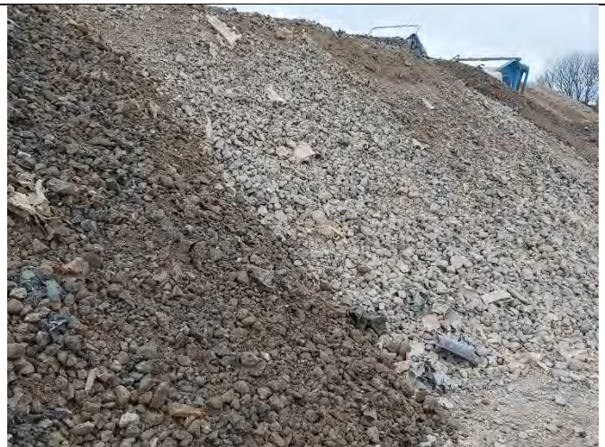
Class 6F5 crushed concrete.
